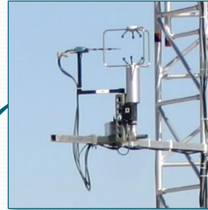
Combo probes located at 2m and 6m
